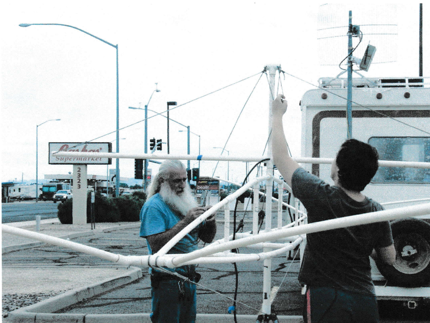
Danuel Quaintance and his grandson Dakota Quaintance assemble a structure to hold a Moxon beam directional antenna.
